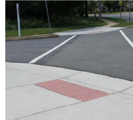
Source Accessible Curb Ramp, U.S. Access Board
