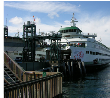
Colman Dock (Seattle) Ferry Terminal
