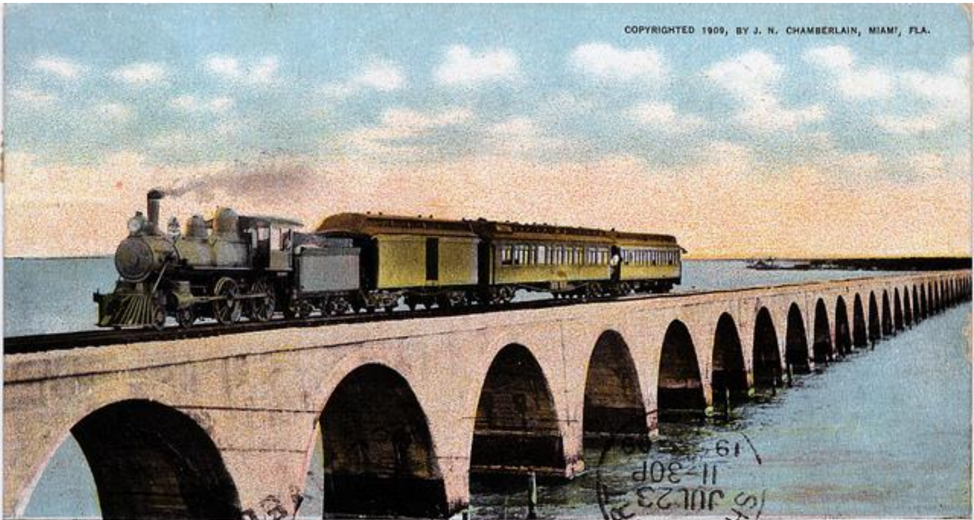
19756 H. M. Flagler's Special, first Train crossing Long Key Viaduct, 2.7 miles long, Long Key, Fla.
