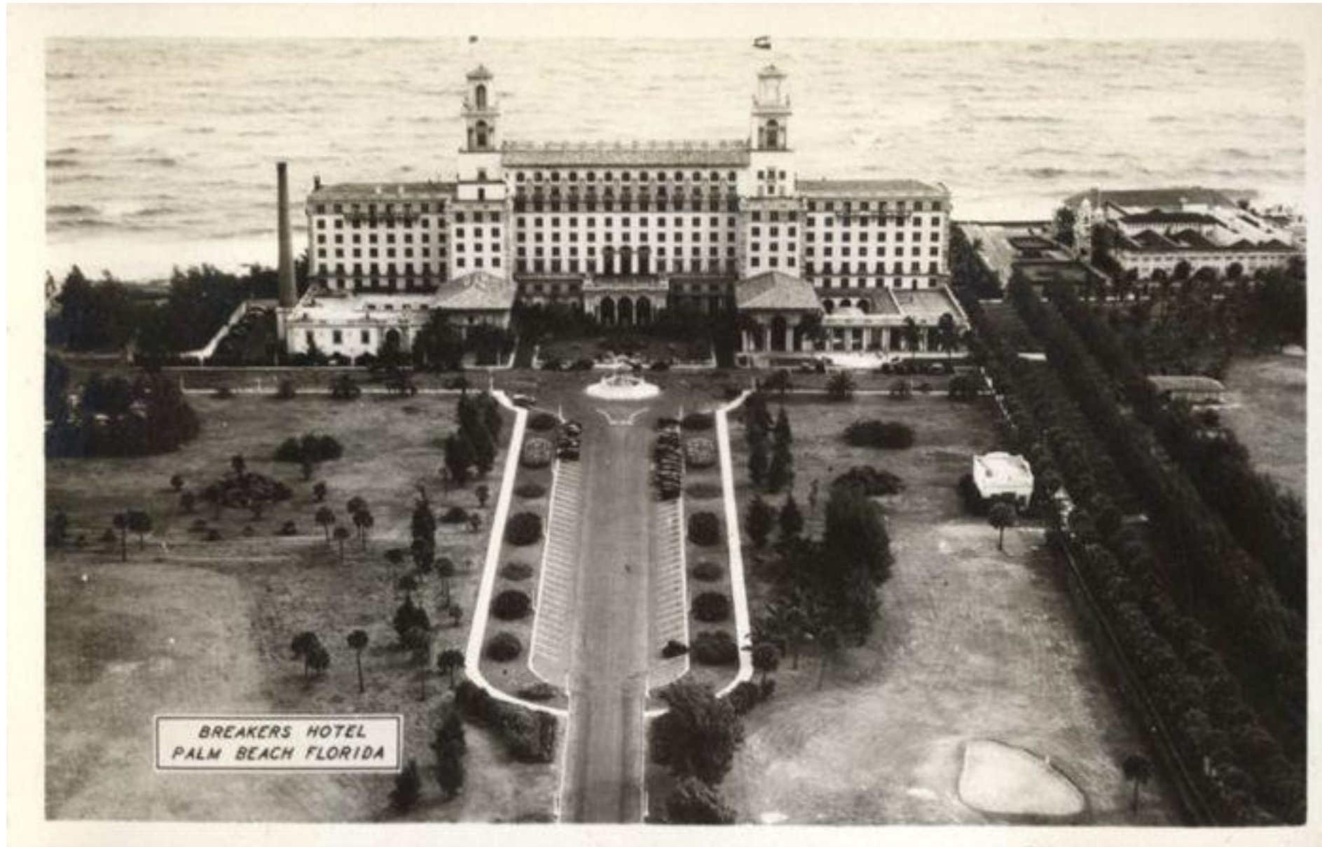
Third and Current Breakers Hotel, Completed in 1926
